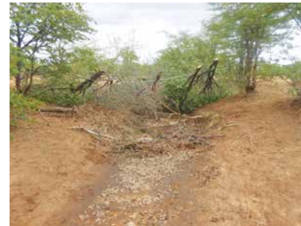
Newly-installed filters to restore a gully in the Kunene Region.
